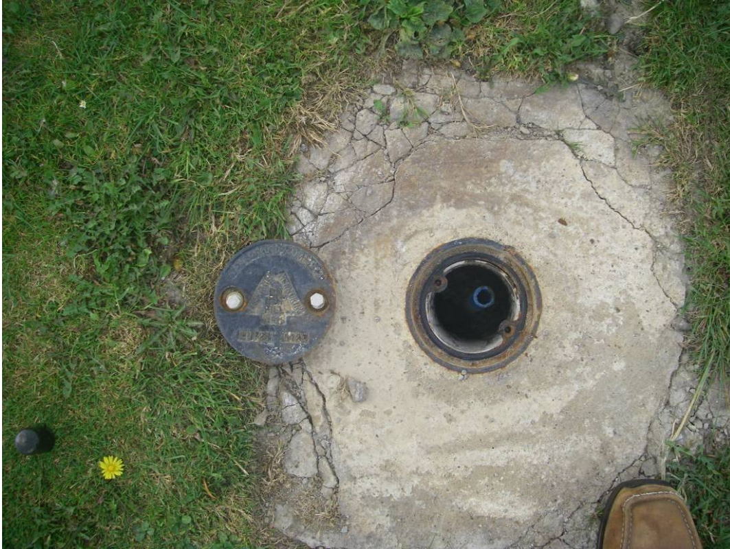
Plate 37 Scarborough South Cliff BH1 Prom
