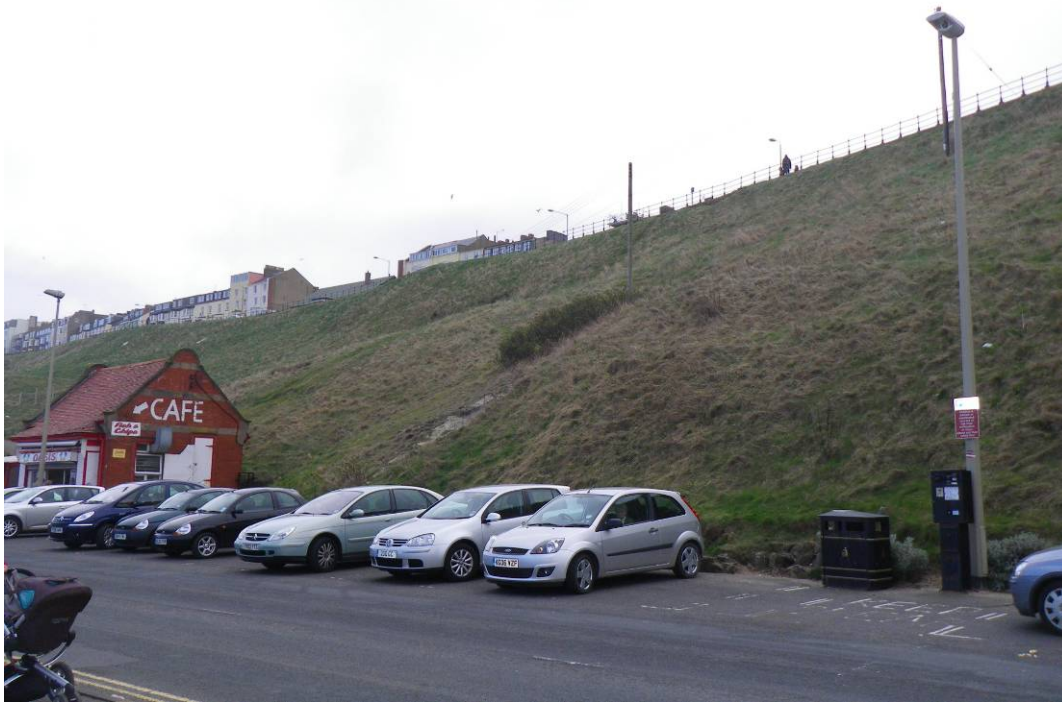
Plate 16 Site view of slopes behind Oasis Café, North Bay.
