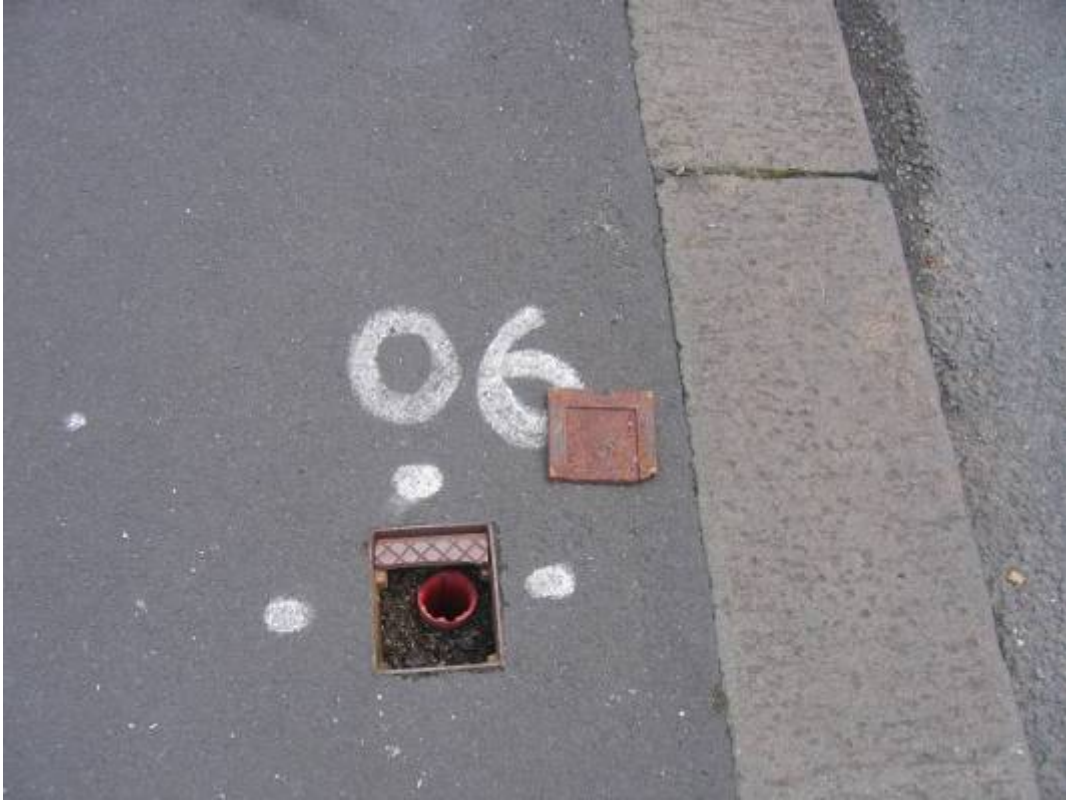
Plate 45 Scarborough South Cliff D1 (AA06)
