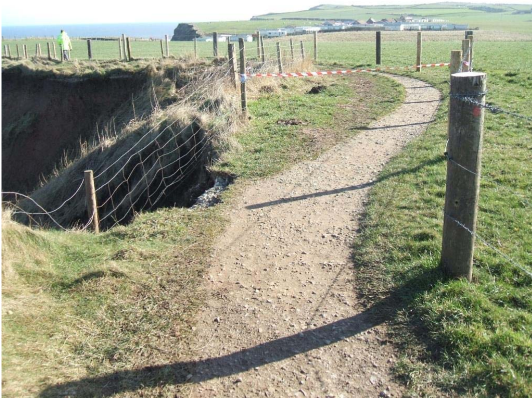
Plate 1 Cliff erosion at Saltwick
