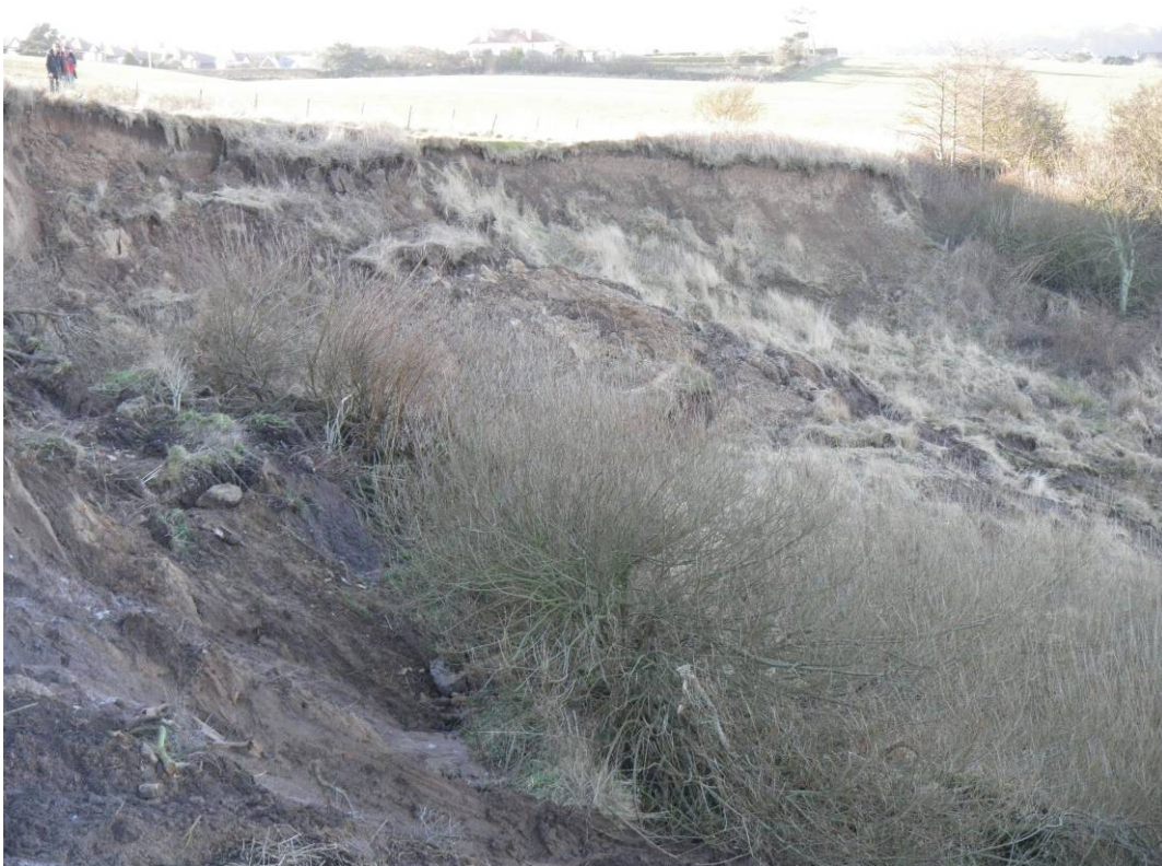
Plate 23 Slope failures on Cornelian Bay side of Knipe Point looking northwest
