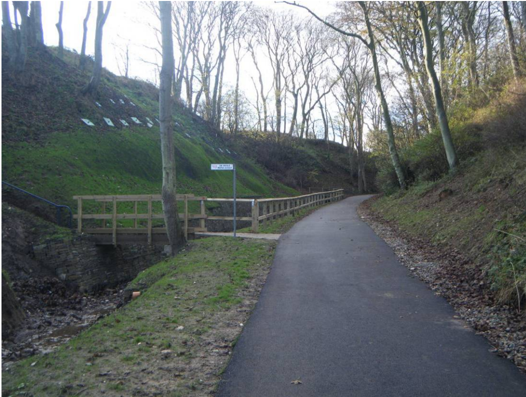
Plate 34 Site view looking up Martin's Ravine. (Remediated slopes on left).
