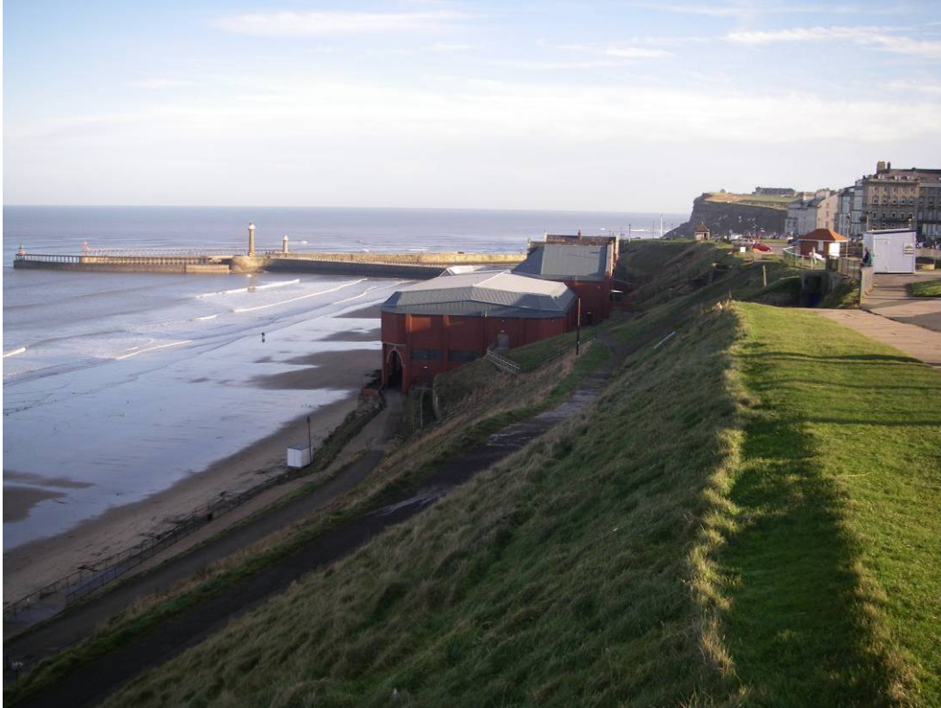
Plate 3 Site view looking east along West Cliff towards The Spa.
