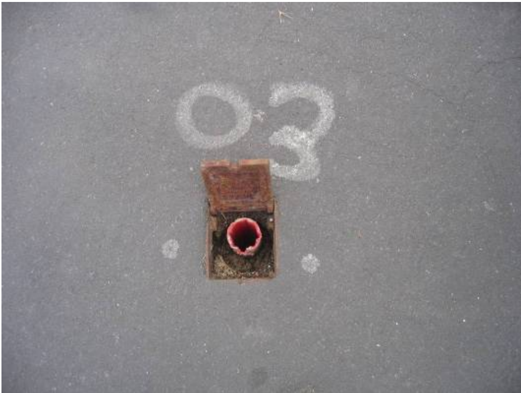
Plate 38 Scarborough South Cliff H6 (AA03)
