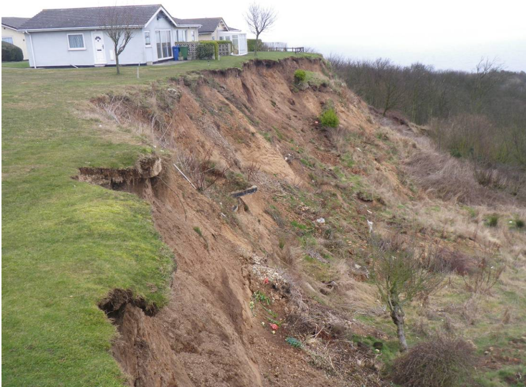
Plate 28 Cliff recession at Knipe Point Headland (8 th March 2010) looking east
