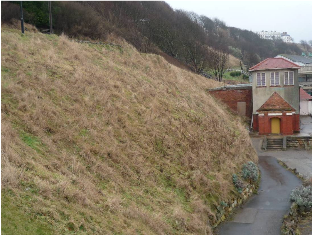
Plate 84 Scarborough South Cliff Slope bulging adjacent the Clock Café (Jan 2010).
