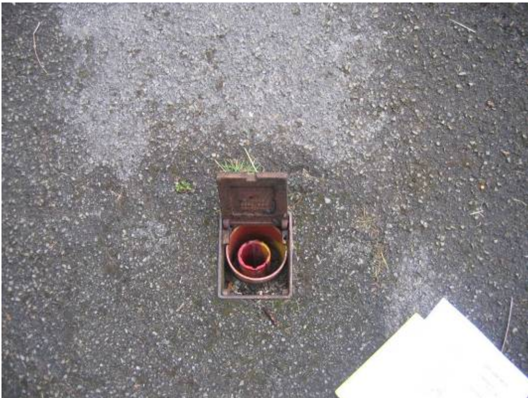
Plate 44 Scarborough South Cliff D3 (AA08)
