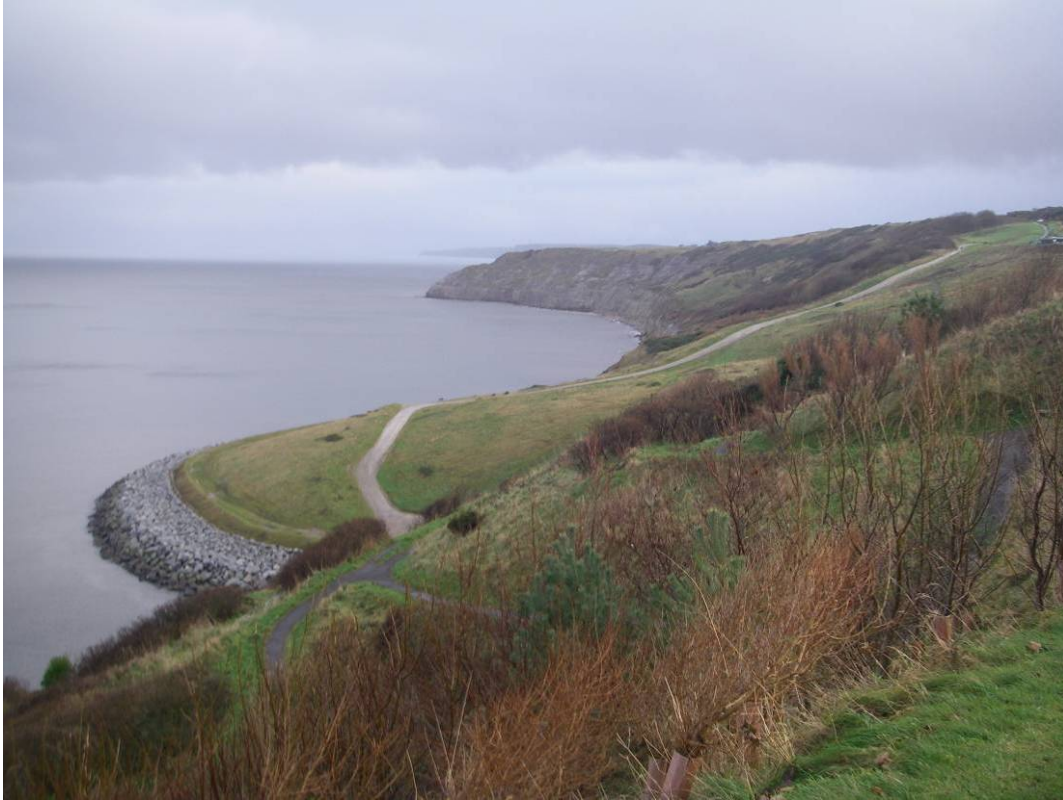
Plate 16 Site view looking south towards Holbeck Gardens and Holbeck Cliff.
