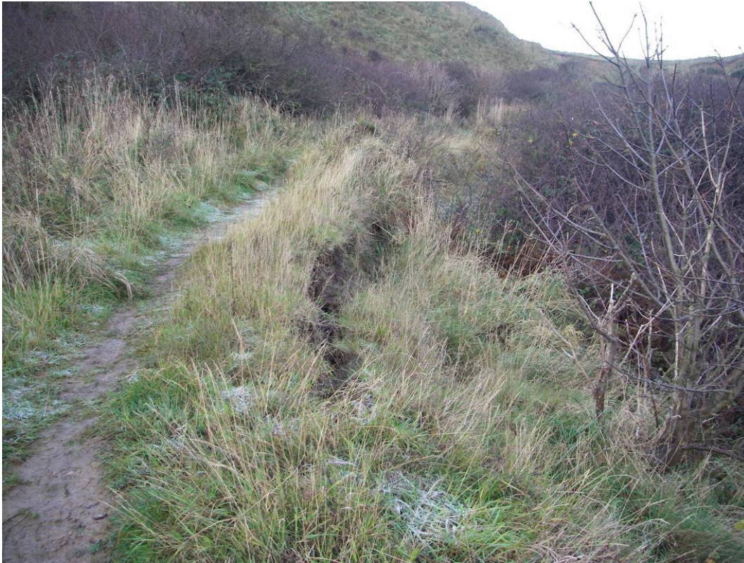
Plate 9 Site view of mid-slope back rotated block and surface tension cracking (November 2008).
