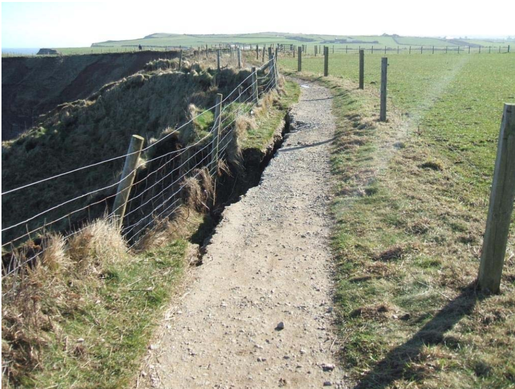
Plate 2 Cliff erosion at Saltwick
