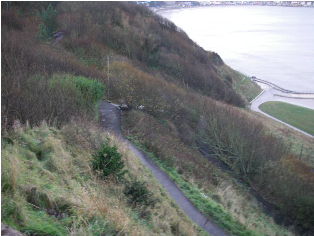
Plate 17 Site view showing steep slope angles above South Bay Pool Cliff.
